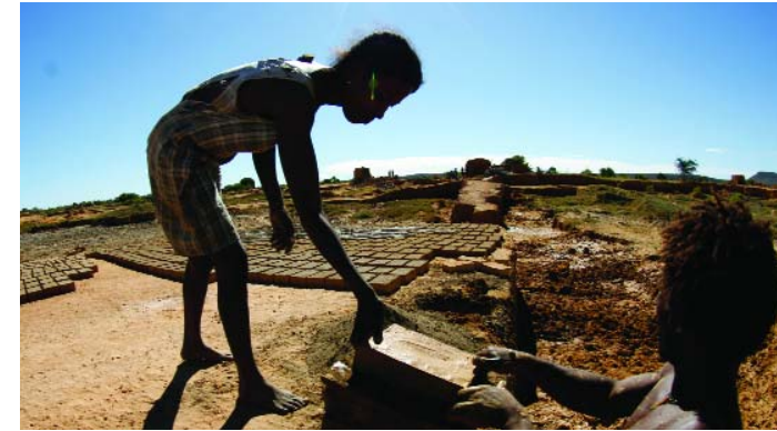
Villagers make bricks for the canteen.
